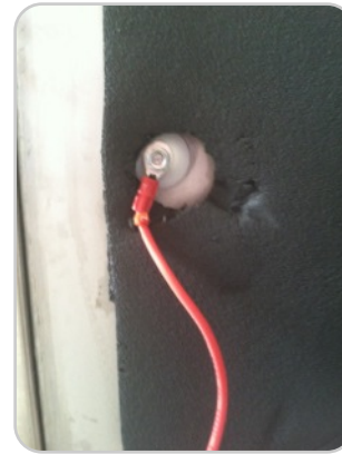
Step 9: Install Re-attach the red wire, outer lock washer and outer nut.
