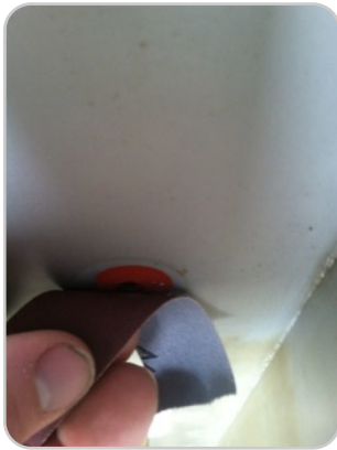
Step 6: Remove old Silicone Use emory cloth to remove any of the old silicone on the tank
