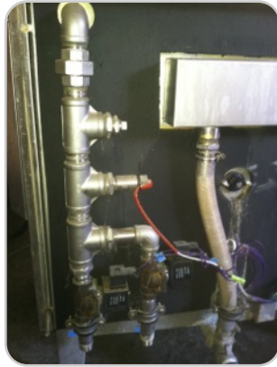
Step 2: Prepping unit Shut off water to unit. Unplumb unit from supply. Remove back panel
