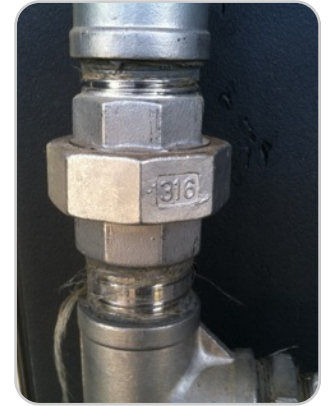
Step 5: Unhook coupler Unhook the pipe coupler and remove the plumbing assembly
