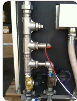
Step 8: Reassembly Reconnect the pipe coupler and mounting clamps. Plug the electrical back in and tighten the screw in the top.
