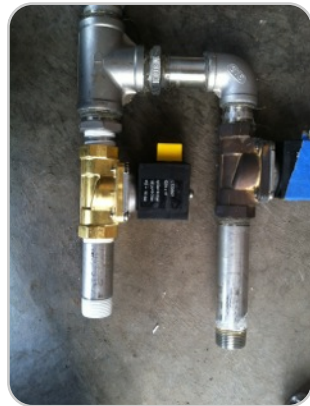
Step 7: Install new valve Install the new valve to the plumbing assembly.
